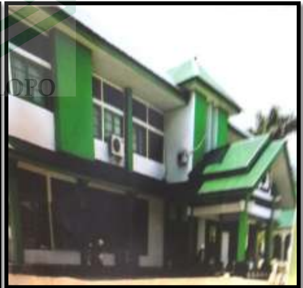
Perpustakaan STAIN Palopo
